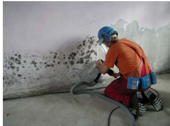
Removal of mouldy wall material
