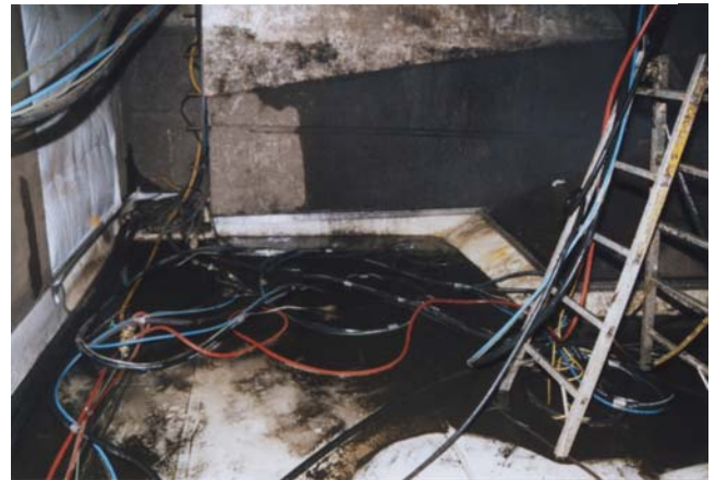
Air supply and breathing tubes in the blast slurry from a construction site involving corrosion protection coatings
