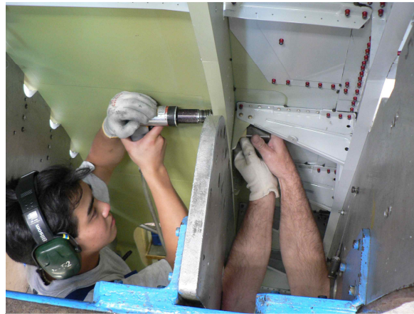
Figure 1.—Use of a riveting hammer and dolly in confined conditions.
