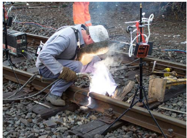
The welding of rail joints
