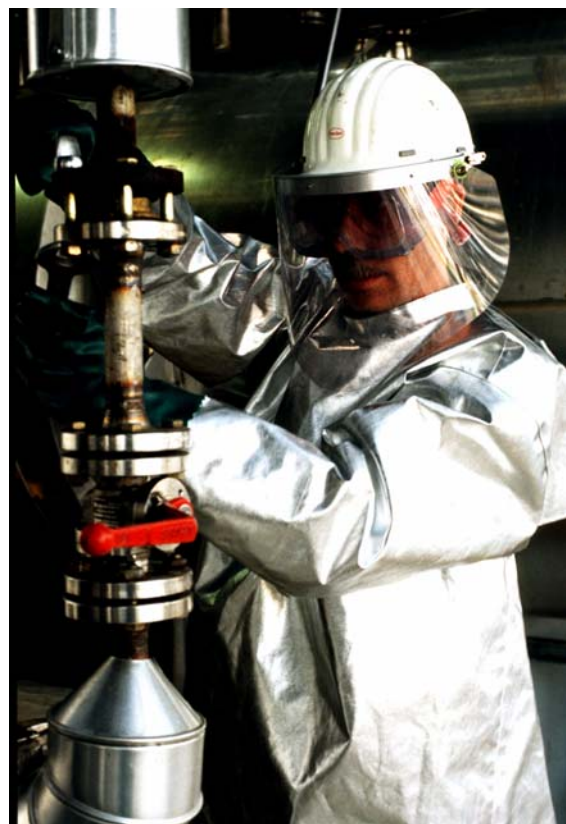
Maintenance/adjustment work with personal protective equipment
